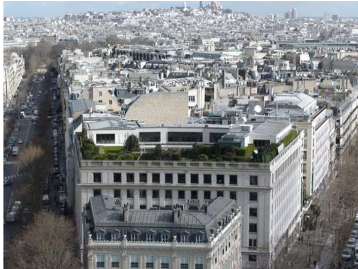
Figure 1.3. Green Roof in Paris, France (Source: sustainablestormwater.org)
